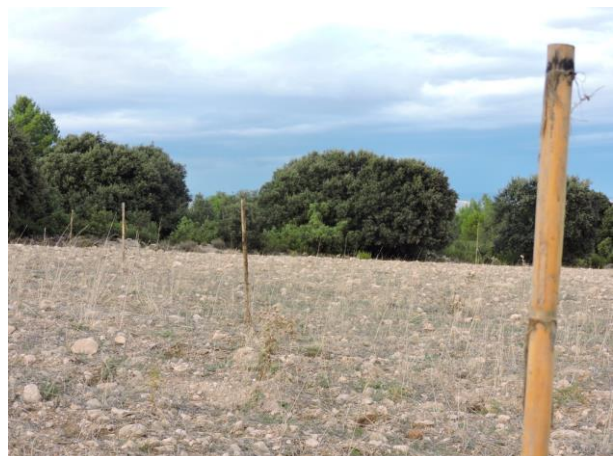
A swale laser is used to place poles to indicate where the swale will be made
